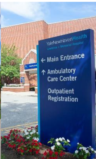
Lawrence + Memorial Hospital
